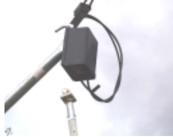
Typical overhead fuse removal and re-insertion
